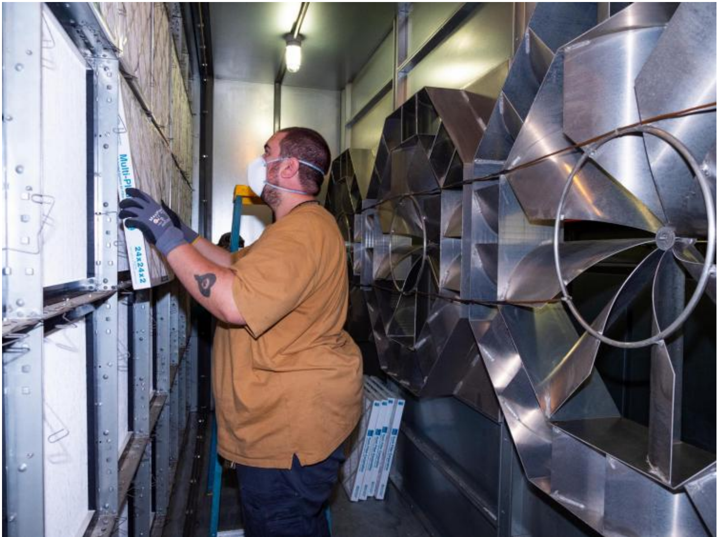
Top: A campus lecture hall with safe distancing measures in place; bottom: Benton Hart, preventative maintenance tech, replaces old air filters in the Indoor Practice Facility with new MERV 13 filters. (Credits: Patrick Campbell/CU Boulder)
